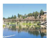
In 2015, a structural condition assessment of the Farewell Bend Bridge determined it needed to be replaced. The bridge is a key bicycle and pedestrian connection of the Deschutes River Trail, linking Farewell Bend and Riverbend Parks.
