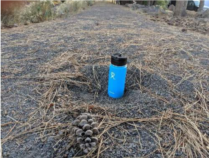
Trail surface aggregate installed by the district in 2017 has poor adhesion and is several inches thick in some locations making trail use difficult.
