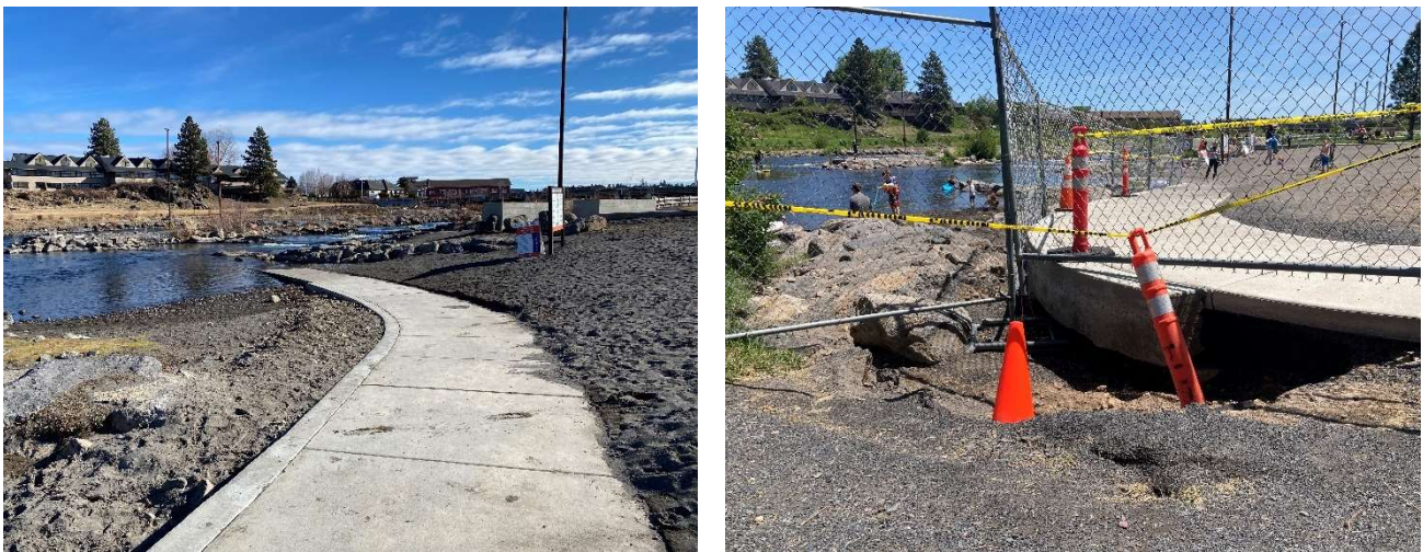
Figure 2. Left: Accessible concrete ramp running through beach to the river, shortly after the new concrete wall was poured. Right: Erosion under and around the path after June 2022 rain event.
