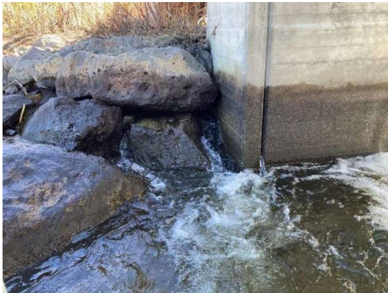
Figure 19. Piping from Habitat Channel to Whitewater Channel
