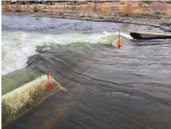
Figure 16. Temporary spacer on static aluminum kickers
