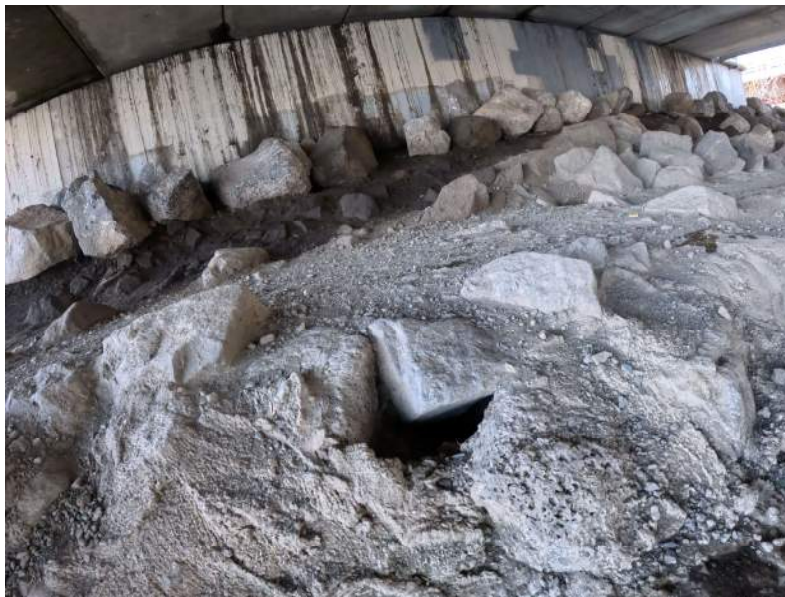
Figure 30. Voids in left bank with piping flows bypassing SP-12
