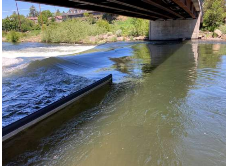
Figure 36. Six large steel gates (11.8' x 4.0') are primary control for upstream water surface. Here two gates are raised on either side of the whitewater channel (June 2024)
