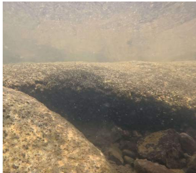
Figure 25. Crest undercut at SP-2
