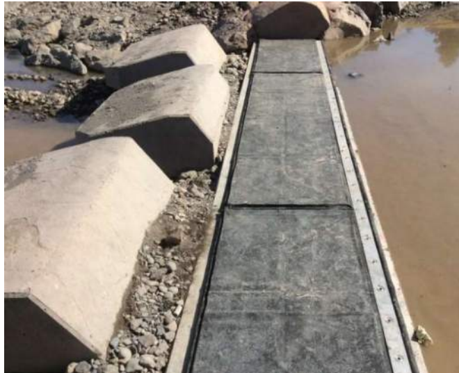
Figure 9. Concrete wave blocks and crest gates during original construction (April 2015).
