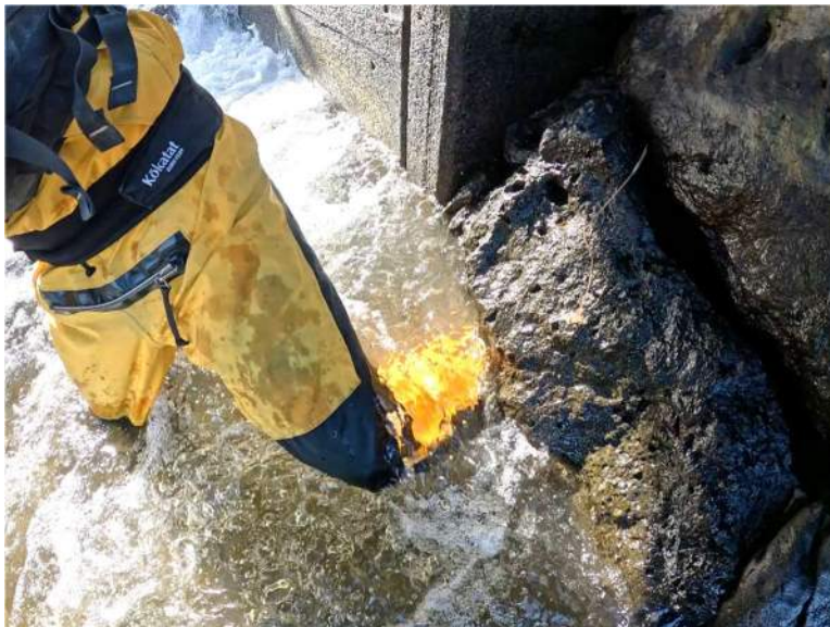
Figure 20. Foot entrapment hazard in void on left side of drop
