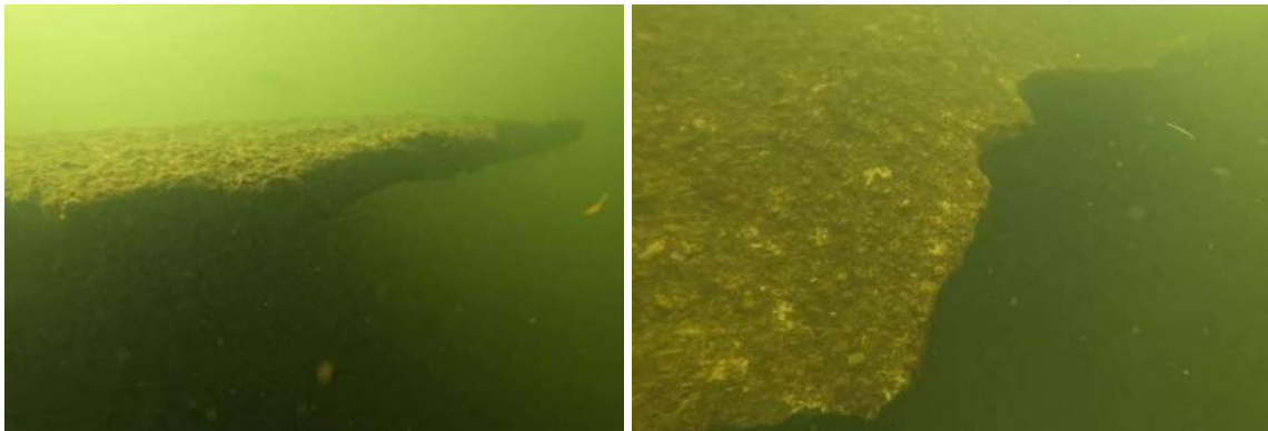
Figure 8. Undercut grout at Jason's Wave exit
