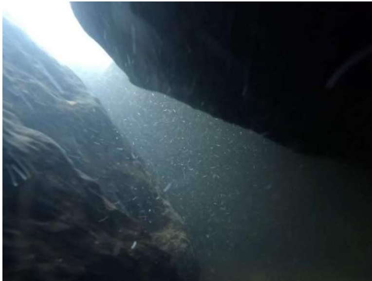
Figure 21. Large voids between boulders in drop structure
