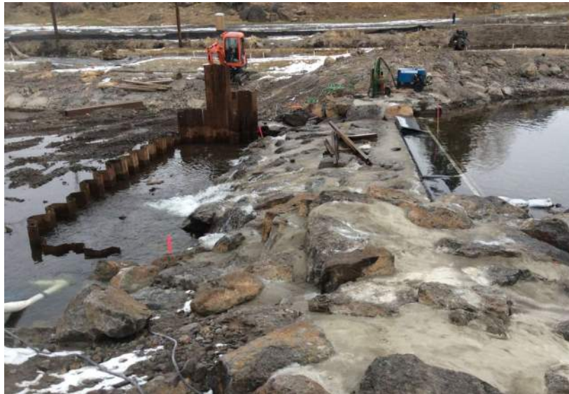
Figure 14. Sheet pile installation during modifications (January 2016)
