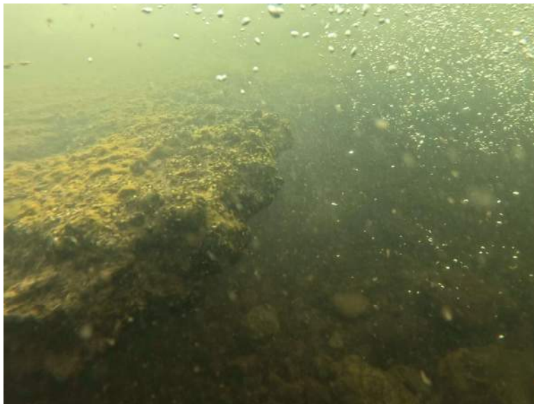
Figure 27. Exit undercut at SP-3
