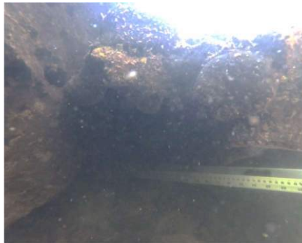
Figure 10. Measurement of upstream undercut Note: Measurement shown is approximately 24" deep
