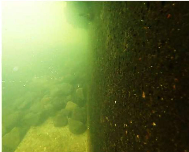
Figure 11. Downstream edge of left wave block and exposed foundation
