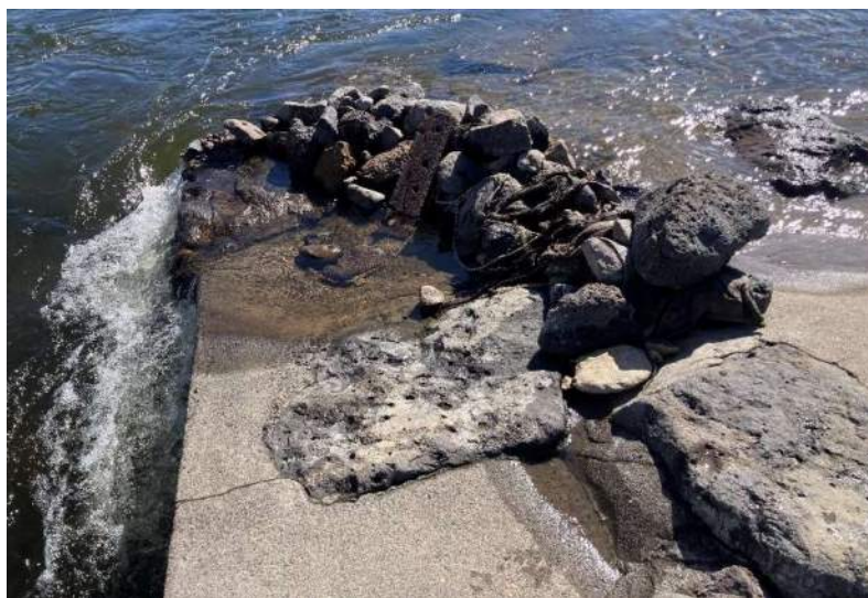
Figure 15. Rock and debris placed on Green Wave wing
