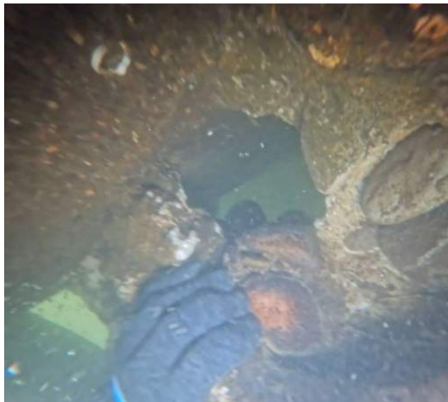
Figure 12. Open hole between scour cave and drop face
