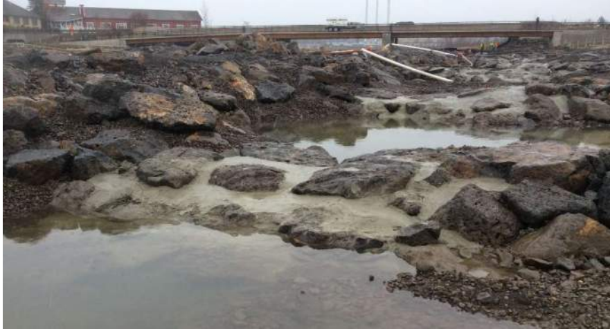
Figure 28. Fish passage channel subsequent to grouting, looking upstream (Dec 2015)
