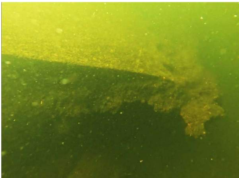
Figure 22. Scour at end of exit ramp
