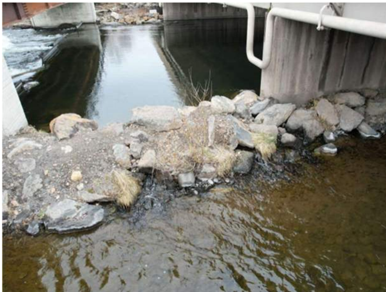
Figure 29. Piping between SP-11 and SP-12 from Whitewater Channel to Fish Ladder Channel.
