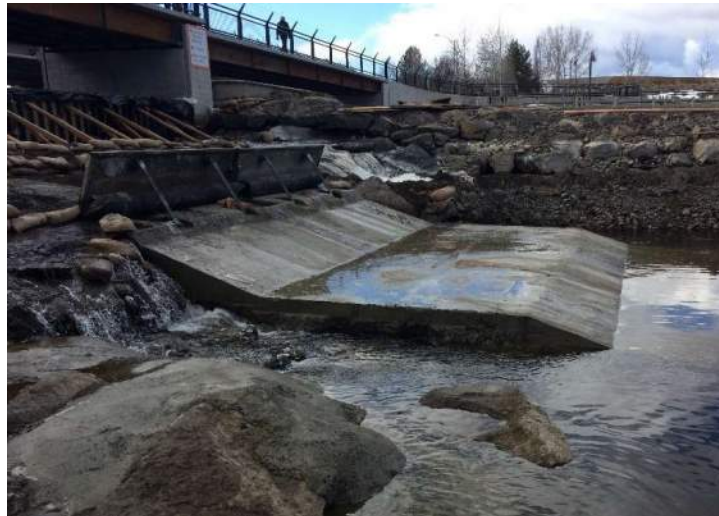
Figure 18. Concrete ramp poured below exit during modifications (February 2017)
