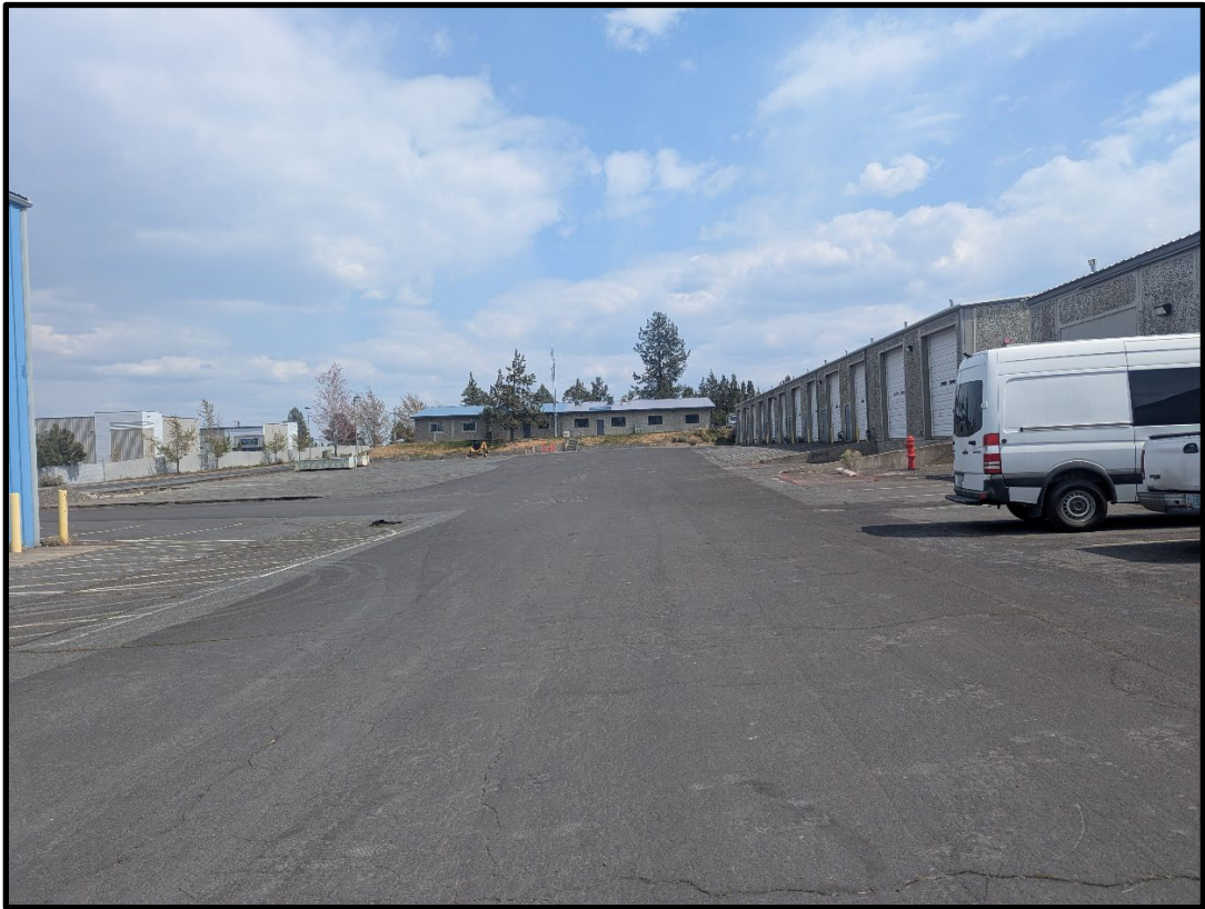
Looking east towards building A
