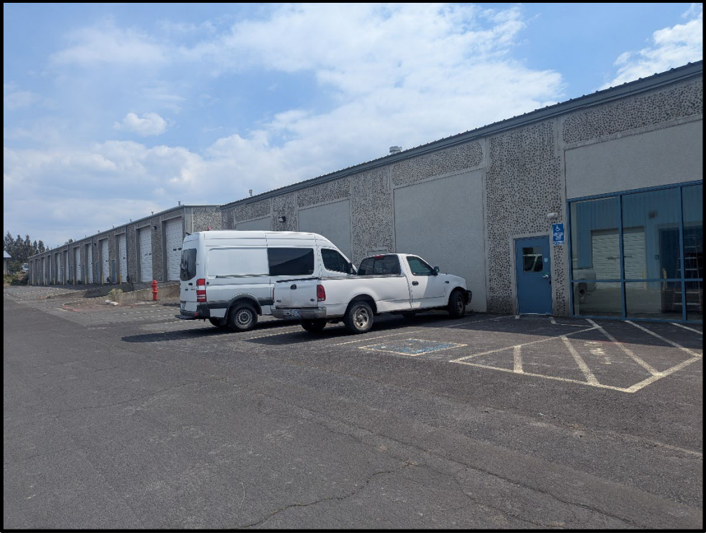
Buildings B and C
