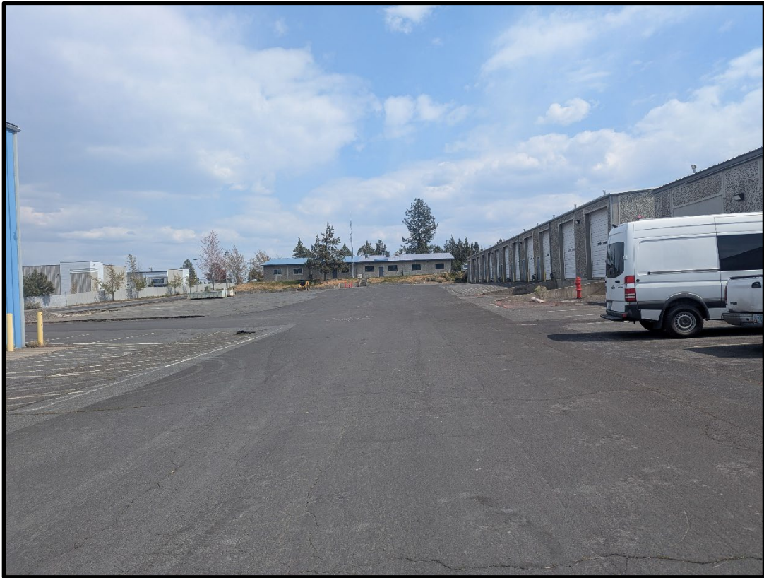
Looking east towards building A
